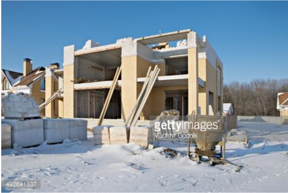
Figure 12: Here is a typical job site, bereft of conveniently placed concrete pillars to mount the scanner on. Time for a good tripod and a tilt compensator.
