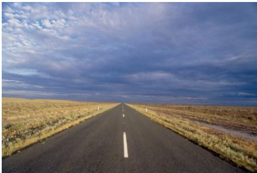
Figure 18: Sometimes the places to mount targets up high are just not available. You can certainly scan a road without a tilt compensator, but getting useful results is very challenging. Cloud to cloud registration here? Forget about it. You would get an answer and it would certainly look right and the residuals would be very small. It might even be right sometimes.
